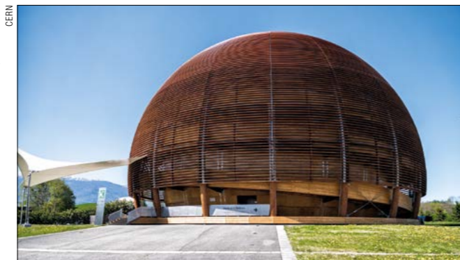
The globe is made almost entirely out of wood (2000 m 3 in total) from Swiss forests, which replenish themselves at a rate of 700 m 3 per hour.
